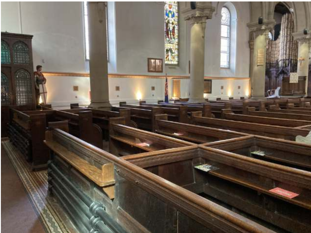
Pews to be removed
