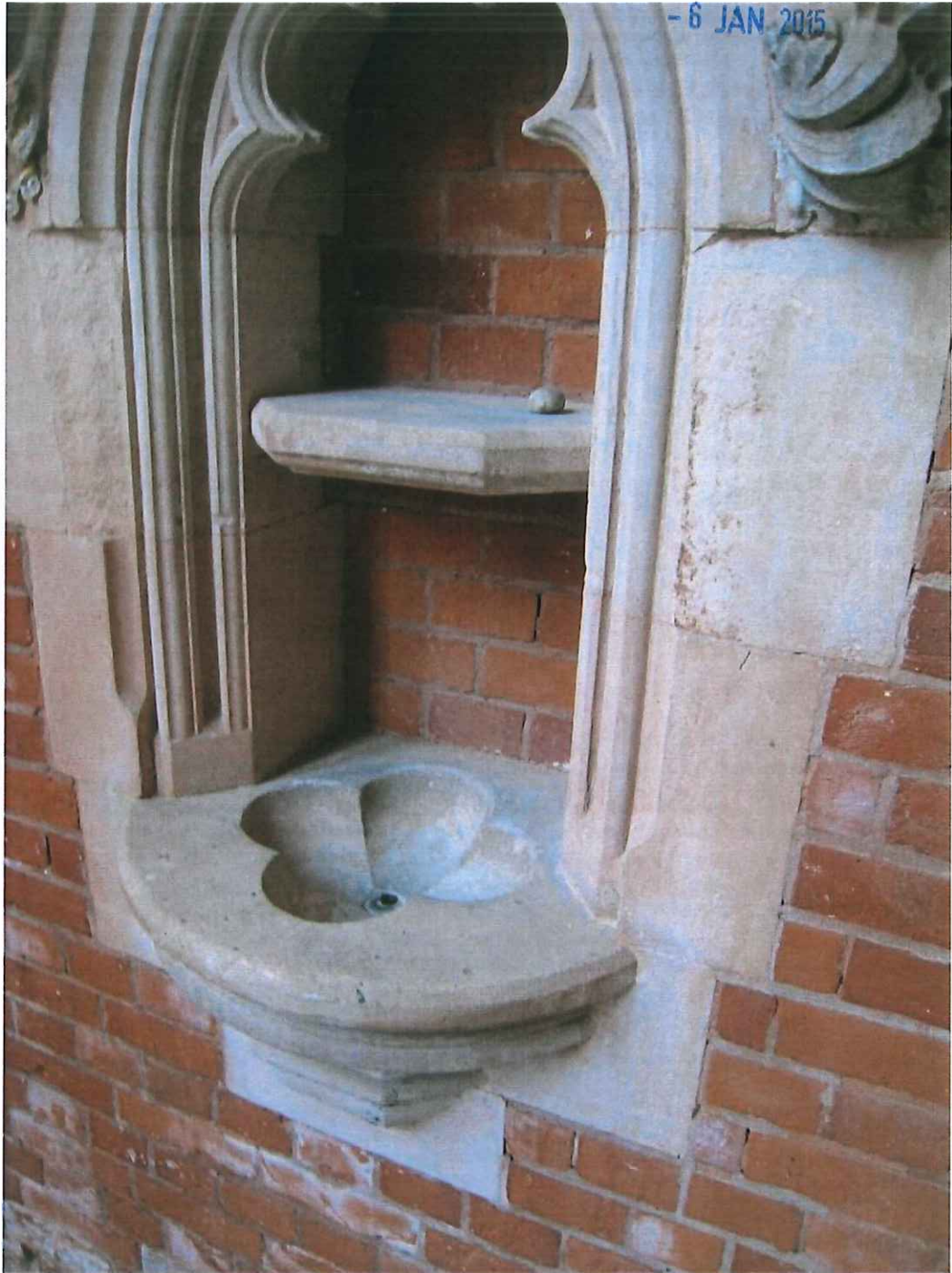
Existing niche (close up)
