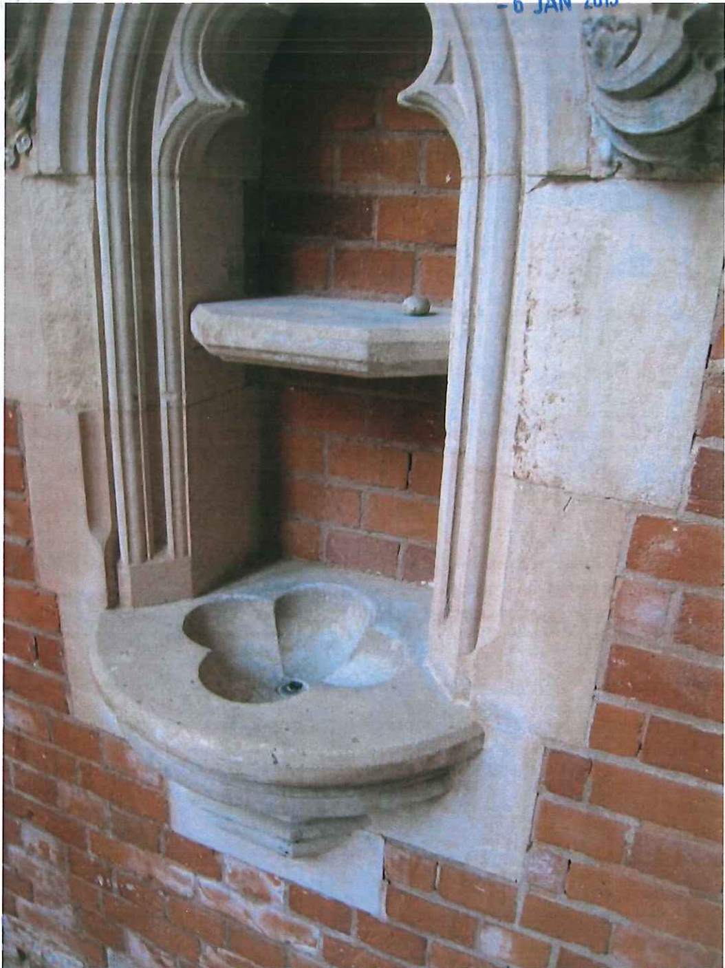
Existing niche (close up)
