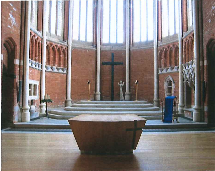
Chancel looking east
