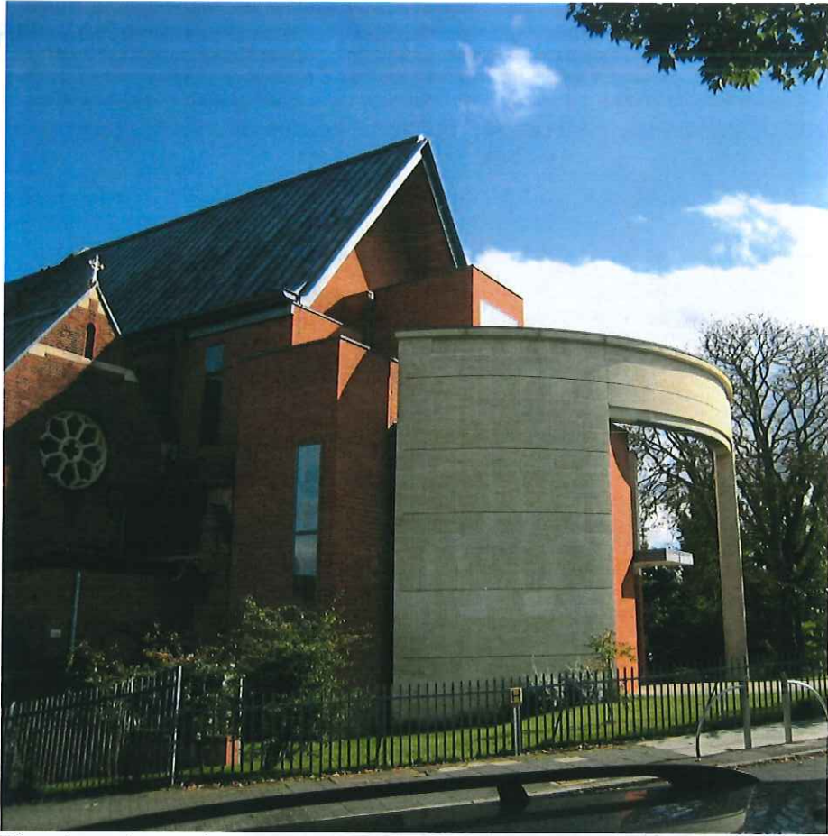
View from the north west.
